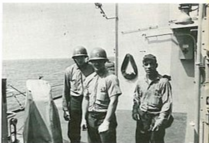
repair party five?
