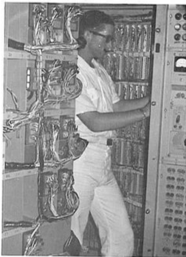
-----and BILBY repairs the damage.
