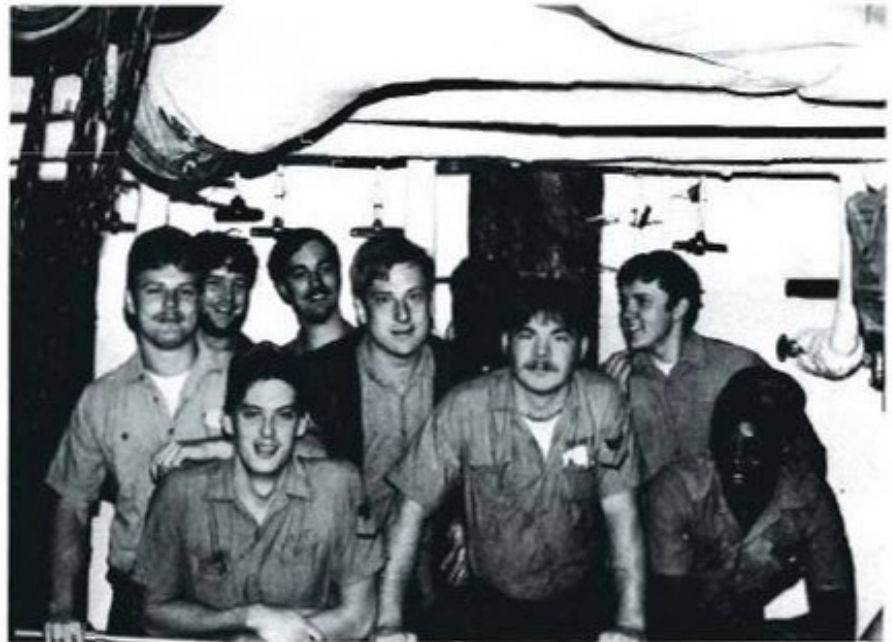
AFT ENGINE ROOM
